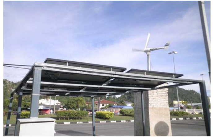
Fig. 4. PV and wind power hybrid generation
